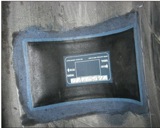
FIGURE 52: Completed Section Repair (Interior View)
